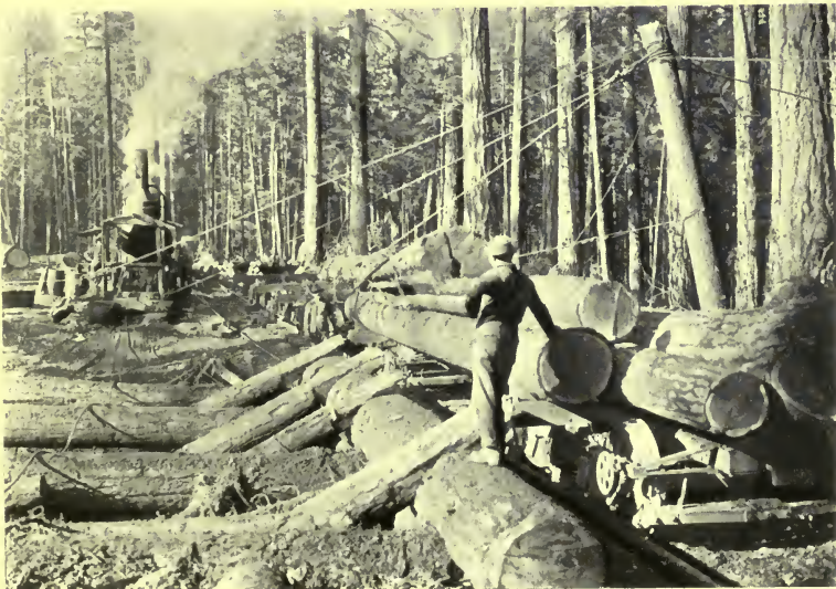
THE DONKEY-ENGINE, "RIGGING SLINGER," AND "GIN POLE" AT WORK
